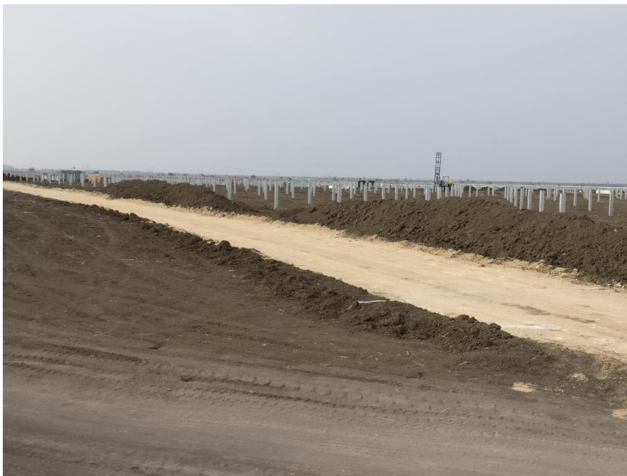
Figure 2-7: View of compacted internal road within the site premises
