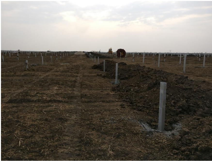
Figure 2-6: View of ongoing Construction at the project site
